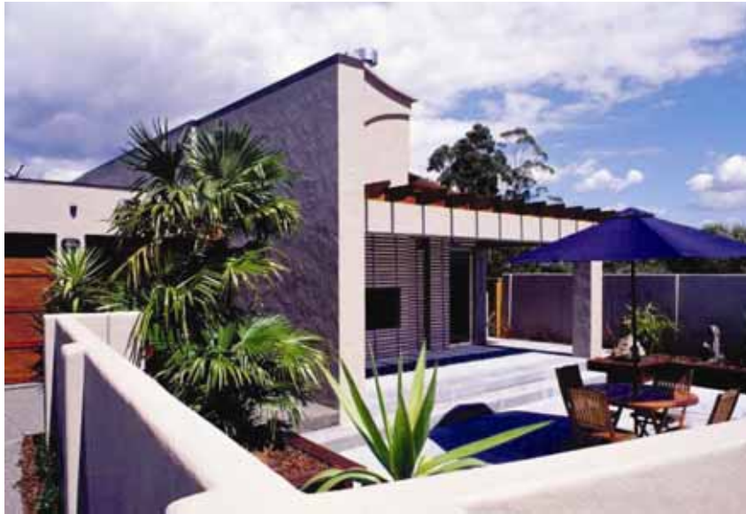
Figure 13 Solid Cladding (Firth masonry)
